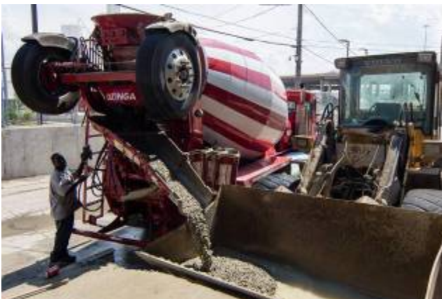
Throwing away top portion of concrete
