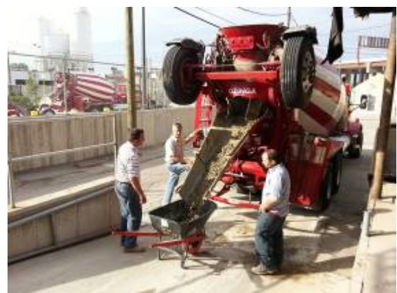
Pouring concrete into cart for sampling
